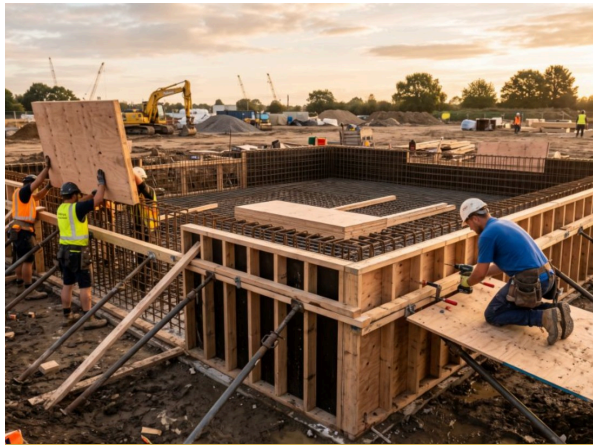
Carpenters and formwork ply. Four pads that all want the gang in the same week.
